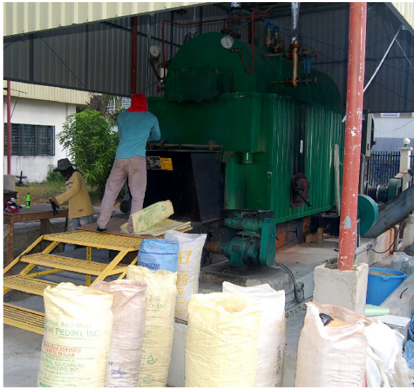
Feeding Rice Husks into the Biomass Boiler
