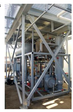
narrowed to inconsequential. The less than 500 lb. anhydrous ammonia charge excluded the system from California's Risk Management Plan requirements. Ammonia is a natural refrigerant and has zero Global Warming Potential and zero Ozone Depletion Potential.
