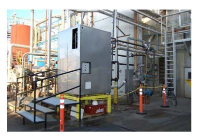
This demonstration unit is designed to supply 75-tons of chilling at the full temperature spread necessary for poultry processing. With a lesser temperature spread, made possible when only "pre-chilling" and "pre-heating" are required, and the existing equipment completes the chilling and heating, then the design capacity increases to 100-tons chilling. Initial operation has been at about 82% of design capacity, and
