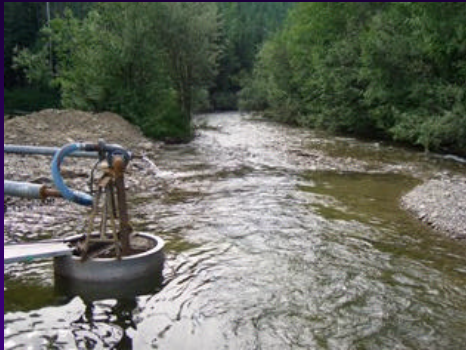
Monument Creek Provides Cooling Water (~40F)
